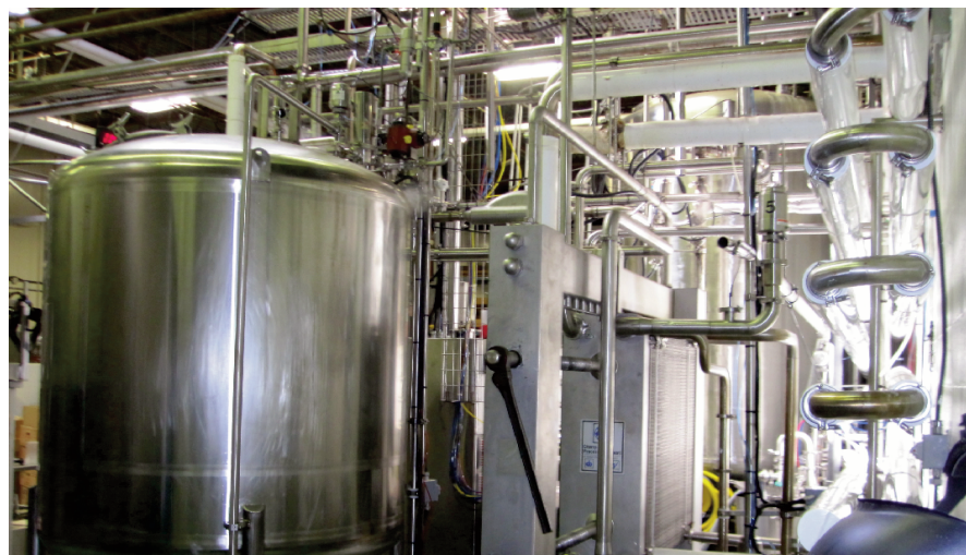
The heat exchanger (center, in the metal frame) quickly cools the mixture of juice and concentrate after it has been Pasteurized.
