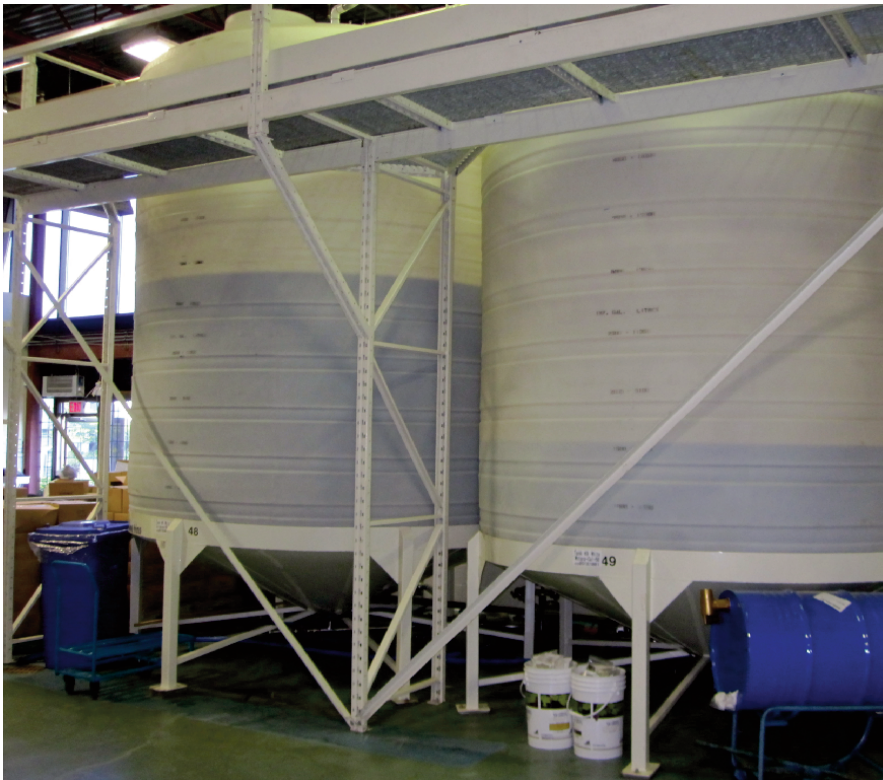
The grape concentrate in these tanks will remain stable for long periods of time due to its low pH and high sugar content. Grape concentrate is blended with juice in wine kits.
